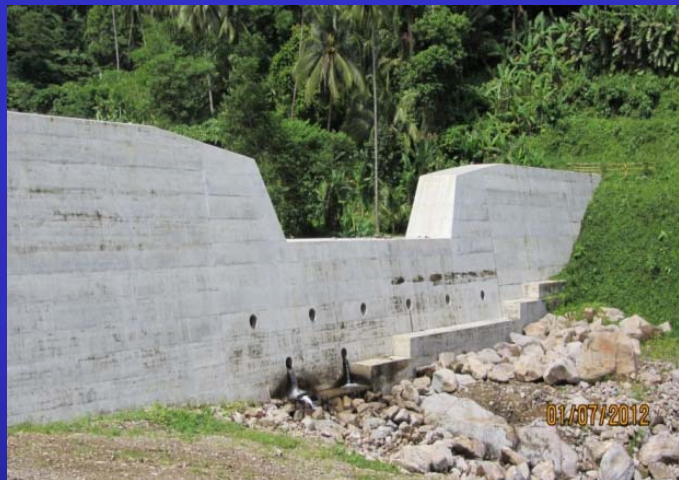
Camiguin Sabo Dam
