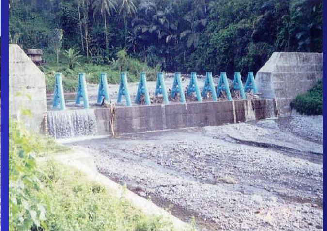
Anilao Slit-Type Sabo Dam
