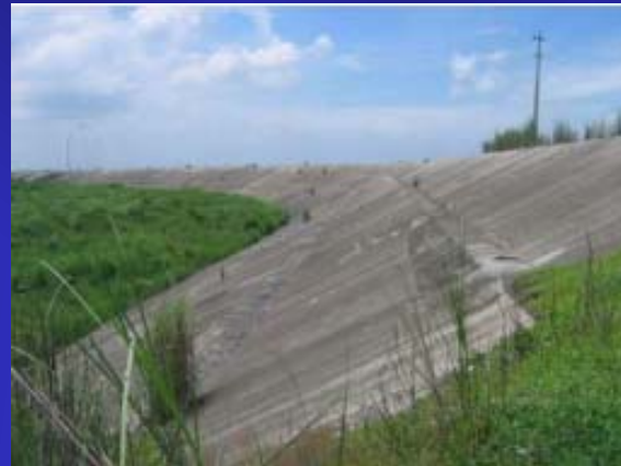
Southwest Mega Dike
