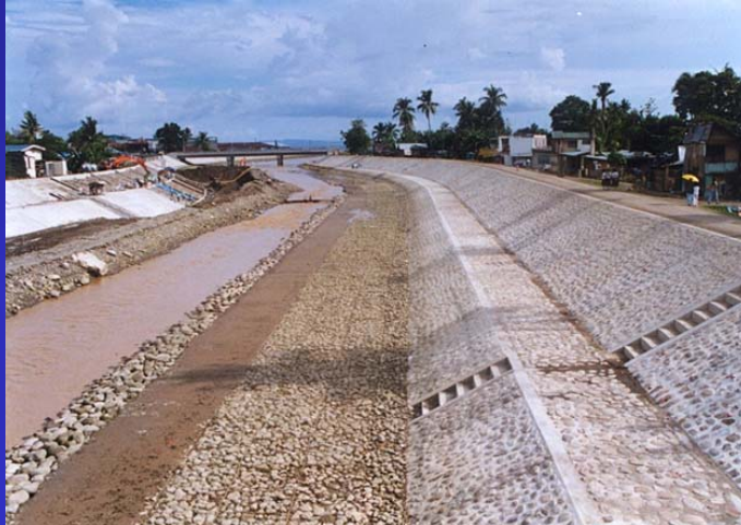
Ormoc Flood Mitigation Project
