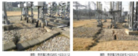
Yorunomori line, Cable in substation (subsidence)
