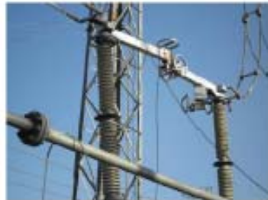
Okuma line 3L, Ground wire (disconnected)
