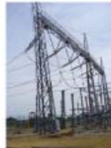
Okuma line 3L & 4L, Steel structure for lead-in (tilted)
