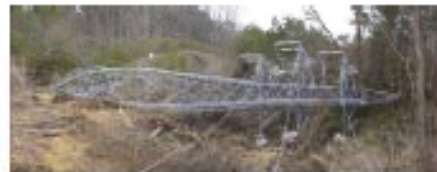
Collapsed tower
