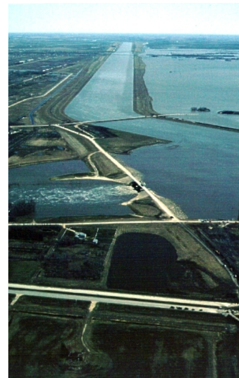
Inlet Structure and Floodway
