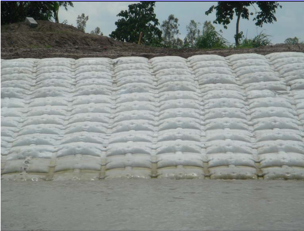
Protection with cement grout mattress
