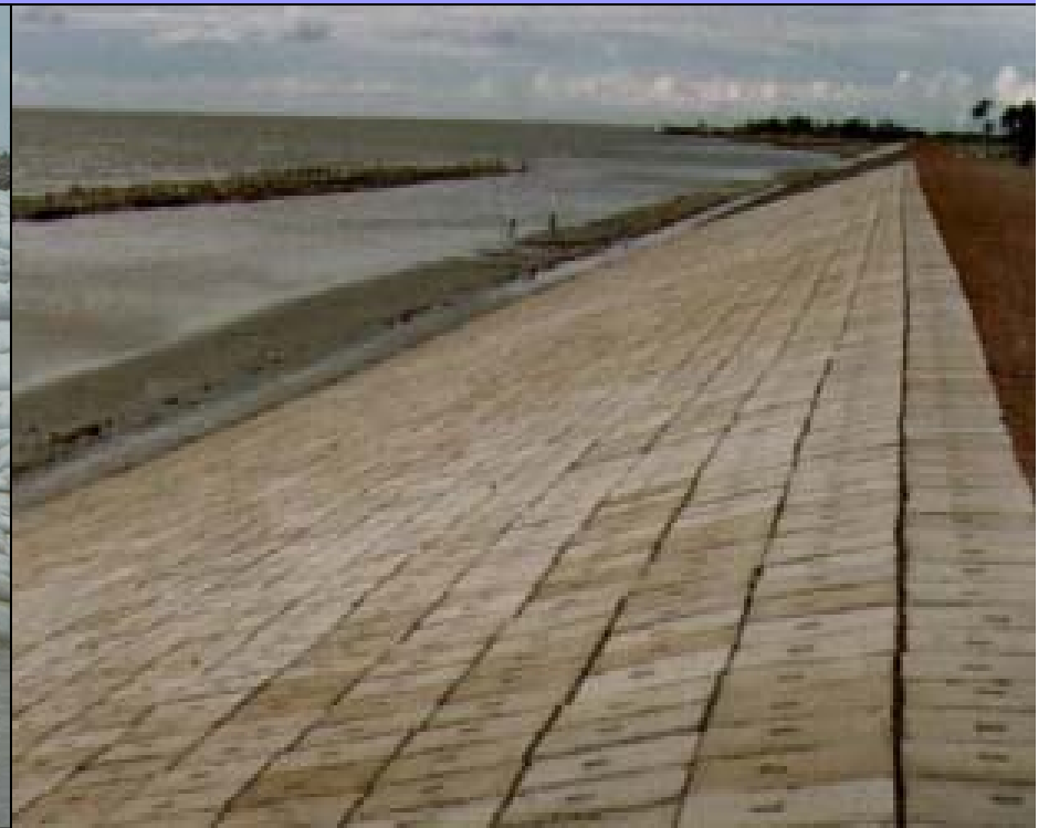
Protection with interlocking cement concrete blocks (tongue-groove type)
