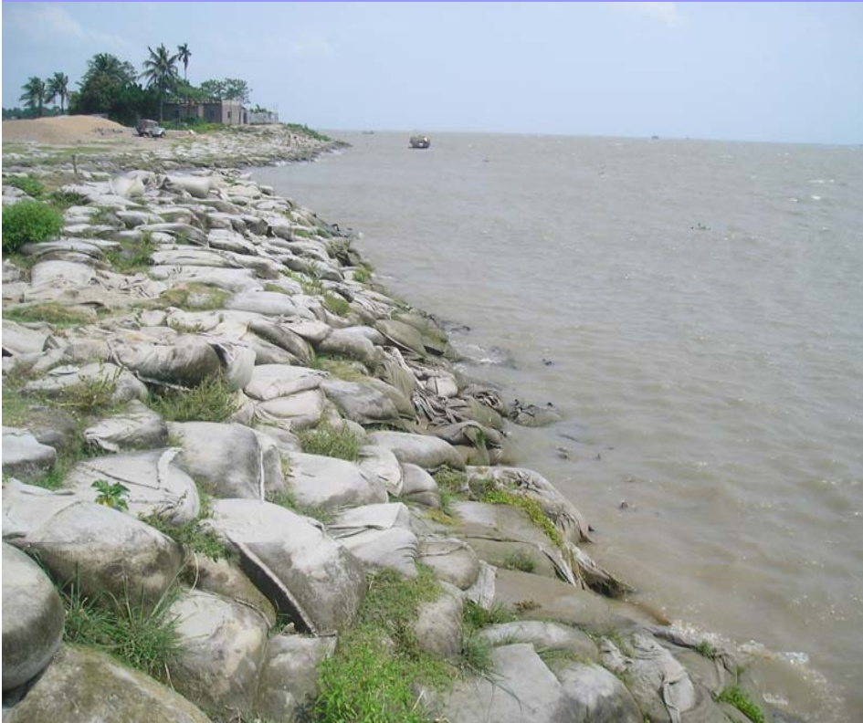
Protection with sand -filled geobag
