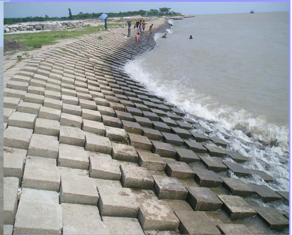
Protection with cement concrete blocks
