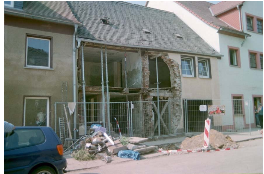
Building type: masonry (clay mortar)
