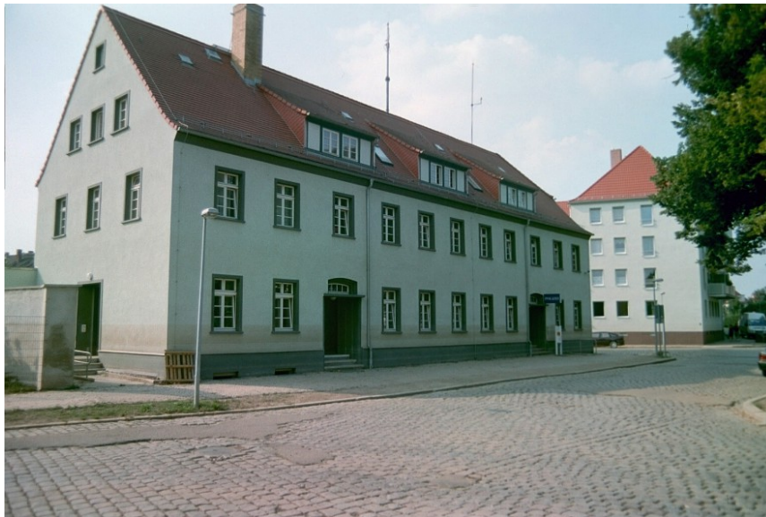
Building type: masonry Damage grade: D2
