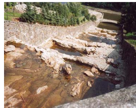
Failure type A: Spillway damages in Saxony (2002)
